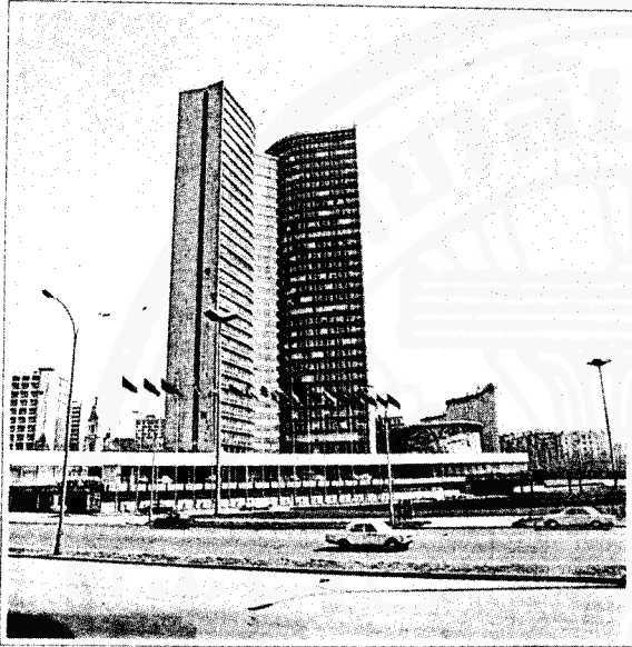
The building of the Council for Mutual Economic Assistance in Moscow
